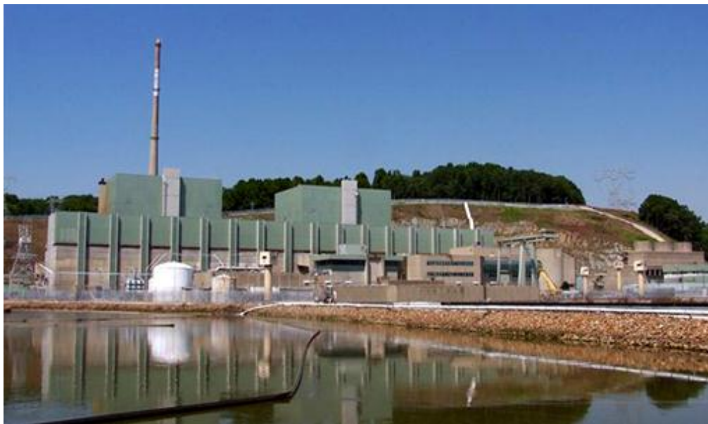
Peach Bottom Atomic Power Station
